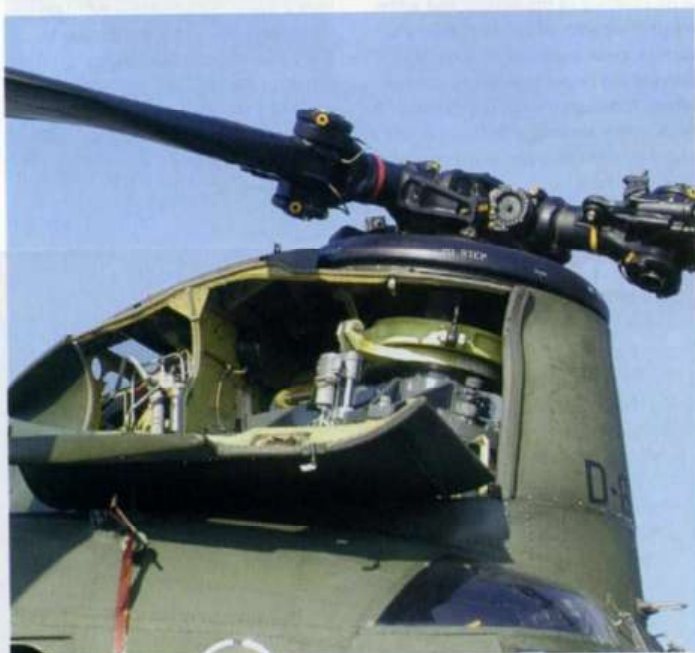
The large hinged access panel and working platform on the starboard side of the front rotor column
