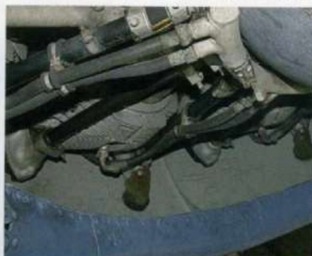
A look inside the cowl, showing the various ignition and oil pipes attached to the engine
