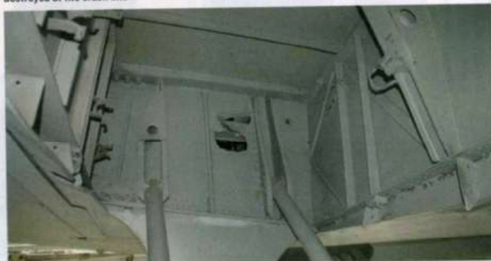
This is the aft bulkhead inside the port undercarriage bay
