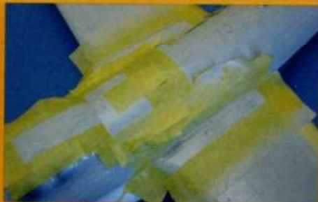
Masking the walkways area
