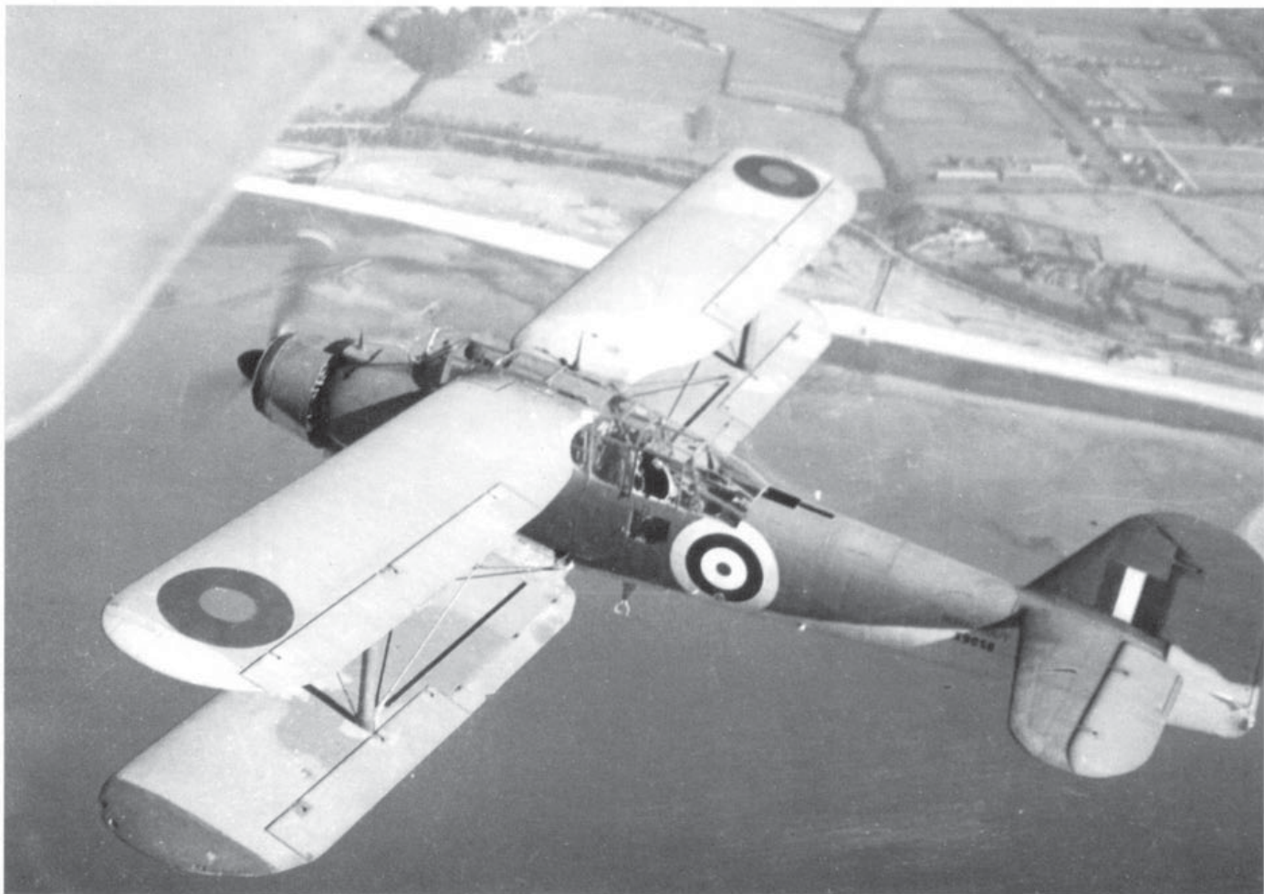
Above: Look at the picture! This appears to be one of an Albacore taking off from a flight deck – but on closer examination a number of things become apparent – the pilot already has the tail lifting, there are two aerials on each outer wing strut and one just below the pilot's cockpit. A compass has been left in its locating hole outside the navigators position. (IWM) Below: Albacore X9058 reveals the shape of the wings and roughly where the camouflage dividing line is. The aircraft was based at Worthy Down at the time.
