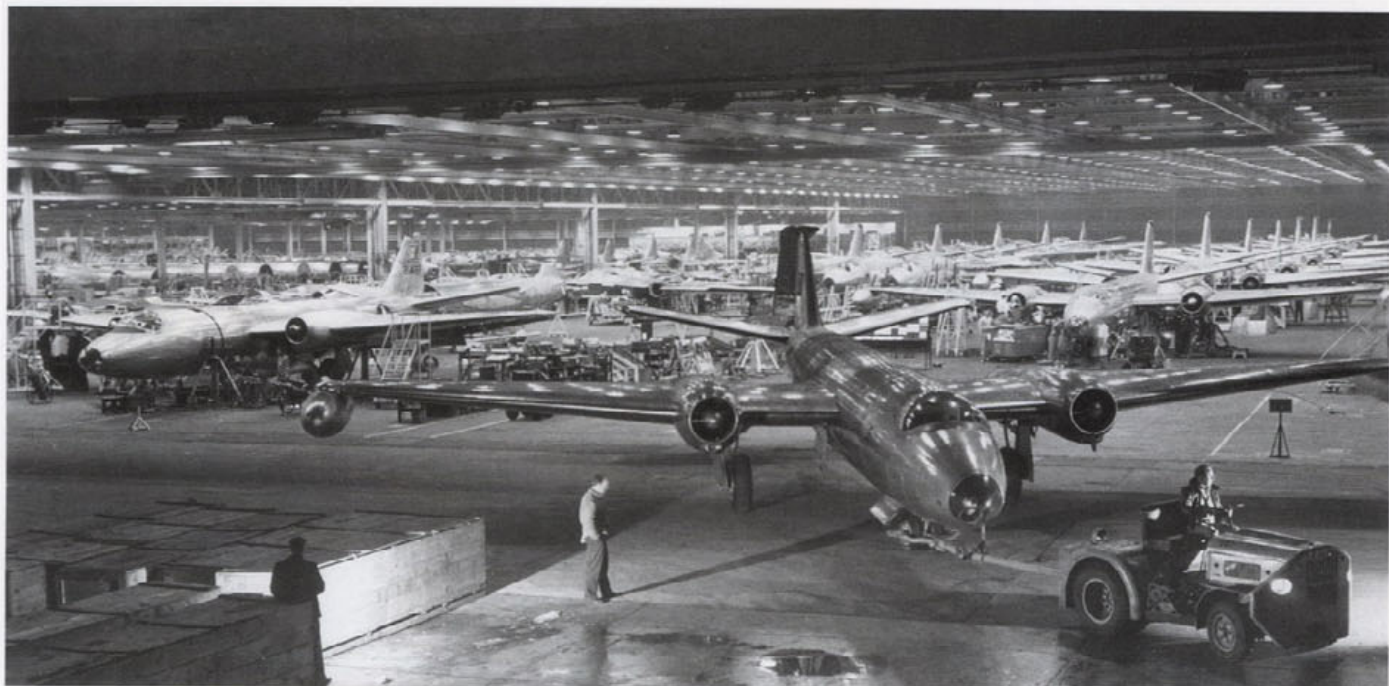
With lines of B-57 Canberras under construction in the background this dramatic night picture shows one aircraft being rolled out for transfer to the paint shop for a coat of gloss black (BBA archives)
