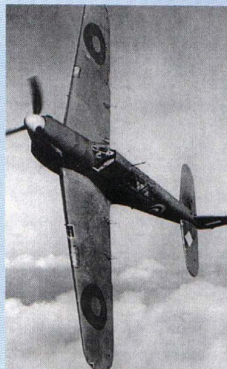
Fifth and final pre-production Fulmar prototype N1858 in 1940. The aircraft is fitted with a trials installation on the wing trailing edge connected to a Fairey-Youngman cruise/dive brake flap. Below: Fulmar Mk.I N1957 of 807 Squadron when based at Worthy Down in 1940 (MAE)
