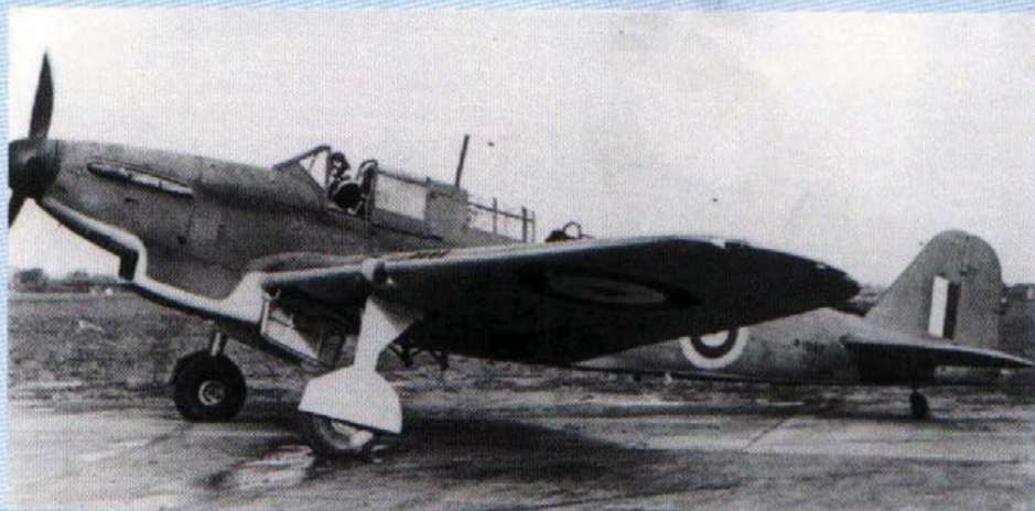
Fifth and final pre-production Fulmar prototype N1858 in 1940. The aircraft is fitted with a trials installation on the wing trailing edge connected to a Fairey-Youngman cruise/dive brake flap. Below: Fulmar Mk.I N1957 of 807 Squadron when based at Worthy Down in 1940 (MAE)
