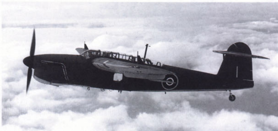
Above: The second prototype Barracuda P1770 which was manufactured with the revised tailplane layout and first flew on 29 June 1941. In all other respects it was the same as P1767. It was allocated to the TRE at Defford where it served from 1942 to 1945 on ASV Mk.II development. (Ian Huntley) Below: Barracuda I P9655 was built at Fairey's Heaton Chapel works in Stockport. Aircraft were moved to Ringway for final assembly and test flying. This photograph was taken in October 1942 and shows the wing fences and torpedo crutches. (Authors collection)
