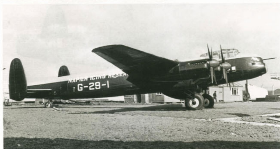
Above: As Napier's Icing Research aircraft, RF342 received civil registration G-APRJ and is seen at the September 1959 SBAC Farnborough Show complete with spray rig and test wing section above the rear fuselage. (Eric Morgan) Left: G-APRJ was later renumbered G-29-1 and then G-36-3 when it went to Cranfield in 1962. (APN)
