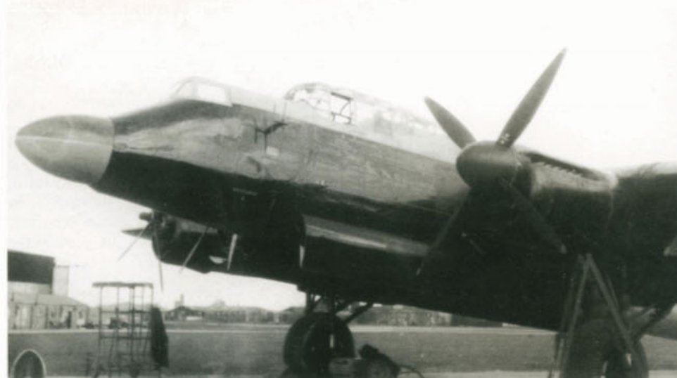
Above: Lincoln RF530 was refitted with a Rolls-Royce Tyne turboprop in its nose and flew in June 1956 registered as G-37-1. It retained its natural metal finish (Bill Harrison) Centre: Lincoln RF533 spent its entire career doing research and received a special nose designed to take all known air-interception radomes. It is seen here at Farnborough in July 1955. (Peter Green) Below: When its active experimental life was completed Lincoln RF533 ended its days with the Stansted Fire School. (Peter Green)
