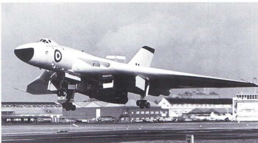
Above: Vulcan B.1, XA894, was used as a testbed throughout its short career. Here it sports the test installation required for the Gyron Junior engine. This aircraft was later used as a trials vehicle for the Olympus 22R engine destined for the TSR.2. It later burnt out on the ground during full power engine runs. (C.P.Russell Smith Collection). Below: The test installation for the forthcoming Tornado engine, the Turbo Union RB.199, seen under XA903 at the 1979 Farnborough air show, (RAE Farnborough)
