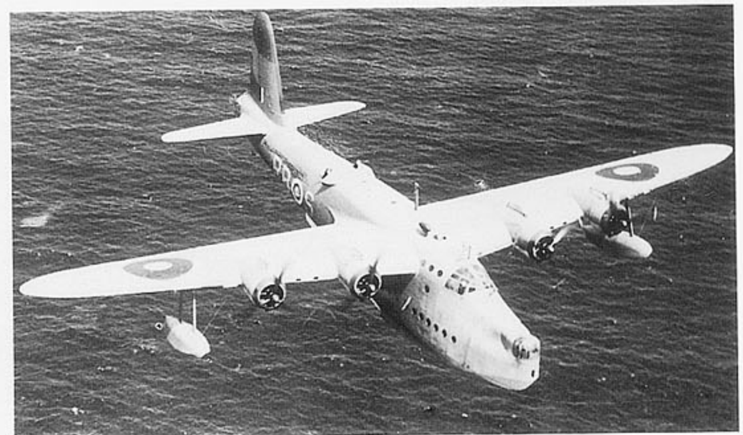
A Mk.I Sunderland displays its slightly swept wings and outward canted engines. A close look at the picture reveals that the censor has blotted out the radar aerials on the rear fuselage and under the wings (MAP)
