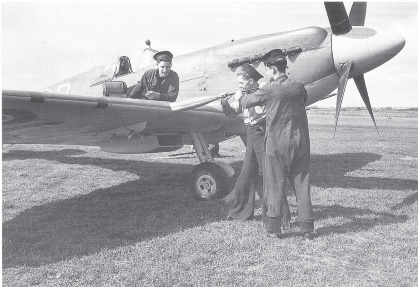
Above and right: Re-arming and refuelling Royal Canadian Navy Seafire F.XVs. These pictures were taken after August 1945 when the first were delivered to 803 Squadron for service on the Canadian carrier HMCS Warrior . Both colour schemes used by the four RCN squadrons are in evidence. (National Archives of Canada)
