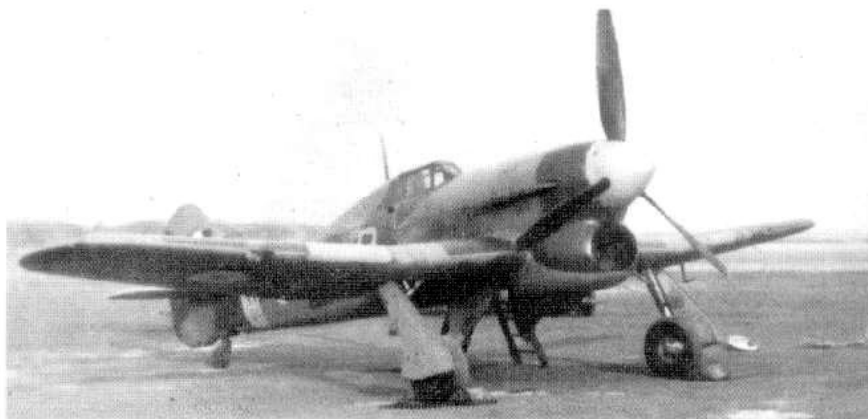
Left: An early Typhoon IA in service with No. 56 Squadron at Duxford late 1941 or early 1942. The machine gun ports in the leading edge of the wing have been covered by doped patches to keep out dust - standard RAF practice. (Public Archives of Canada)
