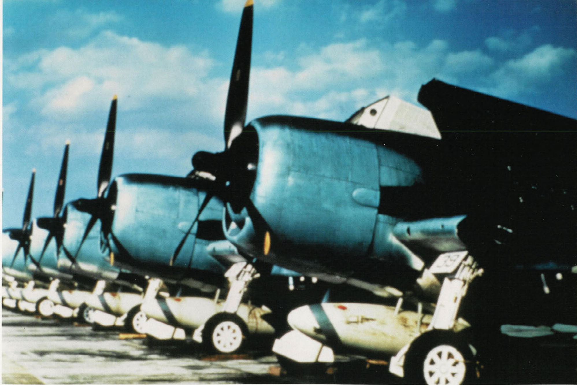
New production F6F-3 line the Grumman Bethpage ramp awaiting delivery. The camouflage scheme was Non-specular Sea Blue, Non-specular Intermediate Blue over Insignia White undersurfaces. All aircraft are fitted with the standard 150 gallon Hellcat underfuselage centerline external fuel tank. Hellcats were built exclusively by Grumman, unlike the Wildcat and Avenger, which were also built by the Eastern Aircraft Division of General Motors. (Tailhook)
