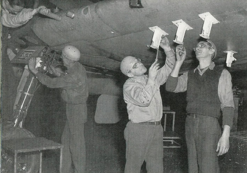
Grumman technicians install zero length rocket launcher stubs under the wing of a F6F-5 (BuNo 79675) on 21 February 1945. The opening above the technician in the foreground is an Amber/Green/Red light used by the LSO to determine if the aircraft was on the proper glide slope for landing. (Grumman)
