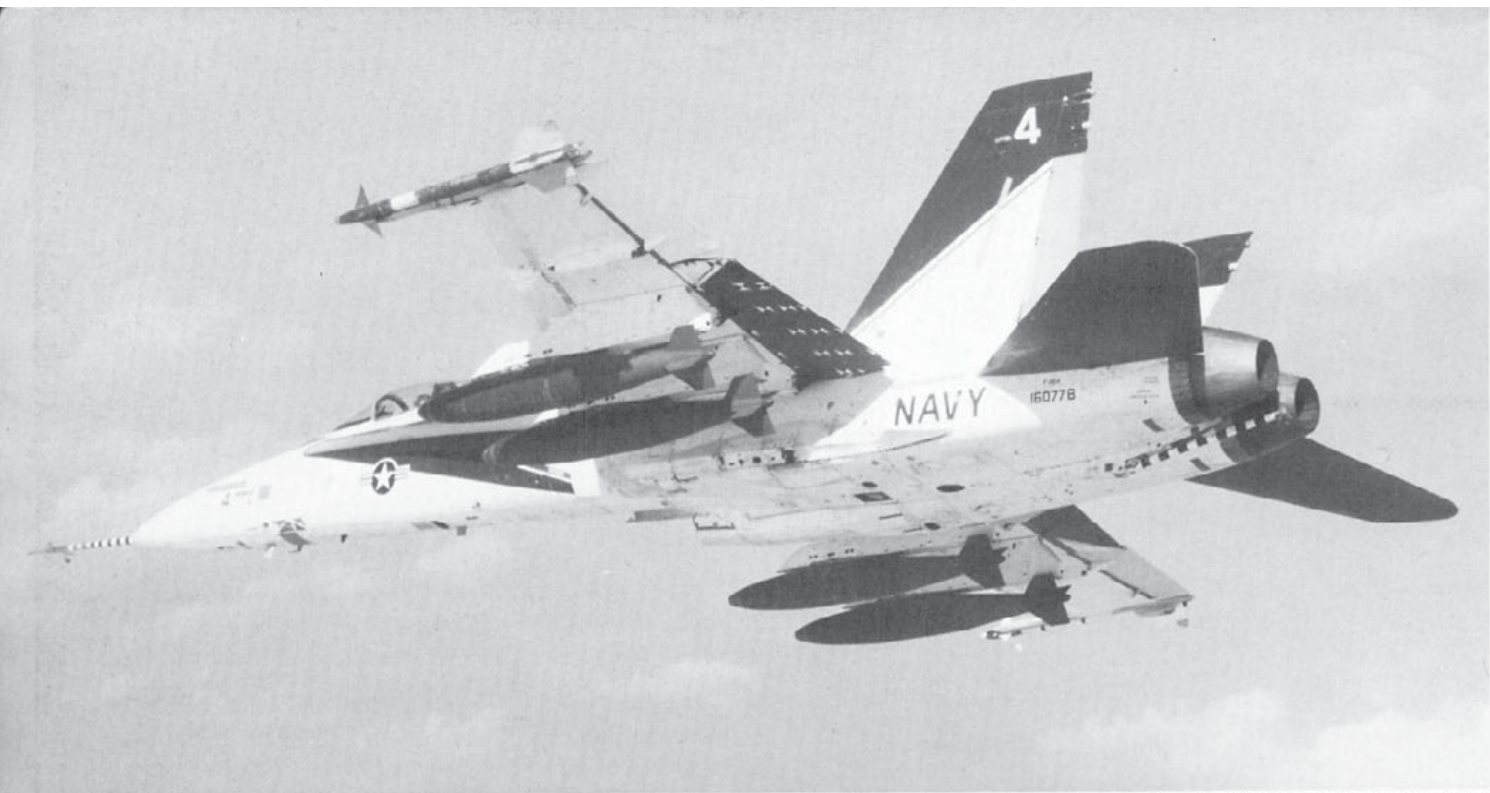
The Number four prototype armed with four Mk 84 low drag bombs. The Hornet can deliver conventional ordnance with almost three times the accuracy of the A-7 Corsair II. (McDonnell Douglas)
