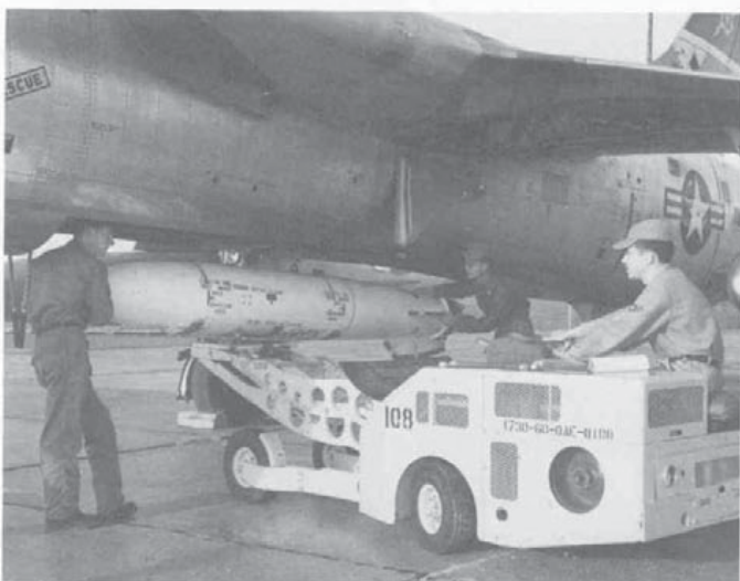
(Above) MJ-1 bomb loader hoisting a nuclear 'shape' into the bomb bay of a Thud belonging to the 335th TFS. (Republic)
