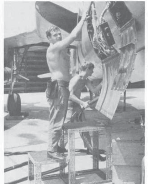
(Above) The six barrel 20mm cannon mounted in the nose of the Thud was capable of firing up to 6,000 rounds per minute, and was effective against MIGs and deadly as a strafer. (Don Kutyna)
