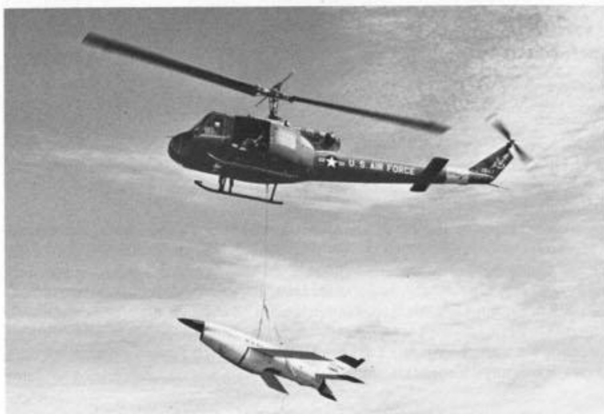
The F model has been used in a variety of roles, including recovery of target drones, in this case a BQM-34A Firebee which had been launched from the Air Defense Weapons Center at Tyndall AFB, Florida in November, 1969. (USAF)
