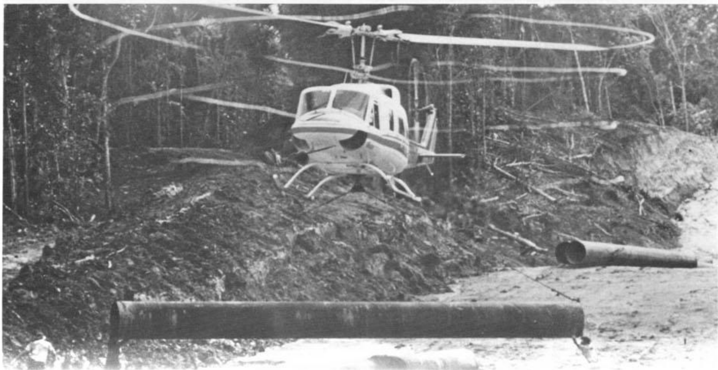
Rocky Mountain Helicopters used their 212 in a pipeline laying job in the jungles of South America, where the twin Hueys power was necessary because of the high density altitude. (Bell)
