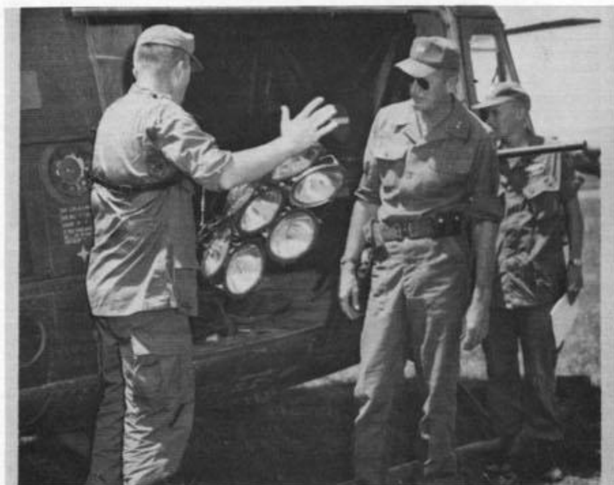
Early in the war it became evident that the good guys would have to find ways to deny the night to the bad guys. This UH-1D mounted the "Lightning Bug" and a 50 caliber machine gun. (Bell)
