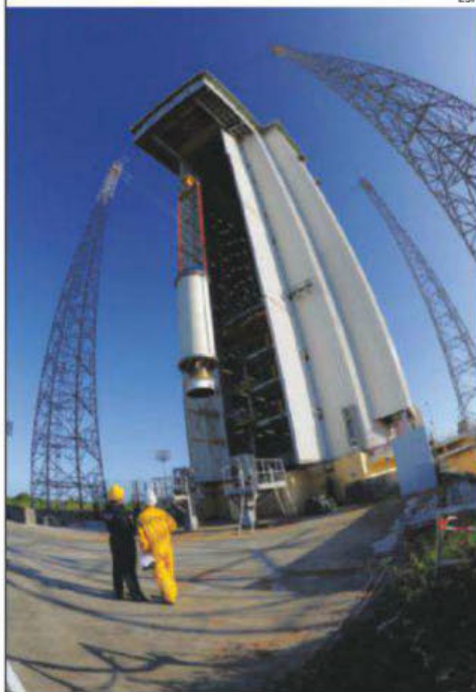
The Vega Zefir-23 second stage is hoisted at the Guiana Space Center in Kourou in preparation for the rocket's February launch debut.
