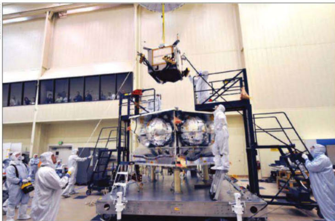
Technicians install the 330-lb. titanium "vault" that will protect Juno electronics from Jupiter's harsh radiation environment. Even with protection, the spacecraft is expected to survive for only a year.
