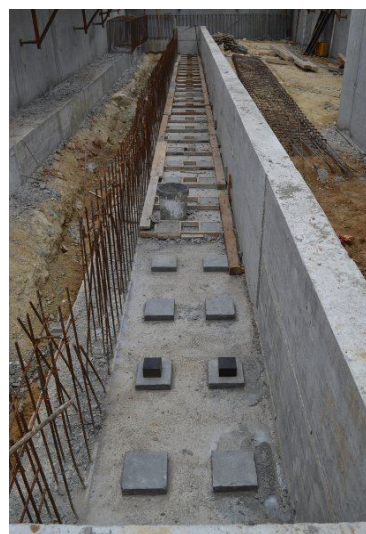
Fig. 4. Current construction status of the shock-tube slab.
