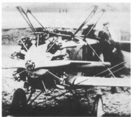
Hungarian Flamingo as a "lighter". Two nose-mounted, 8-mm machine-guns are clearly visible in this view of the locally-built Hungaria Variant V which was a basic lighter-trainer. (Photo: Aero Archiv Winkler-Budapest)
