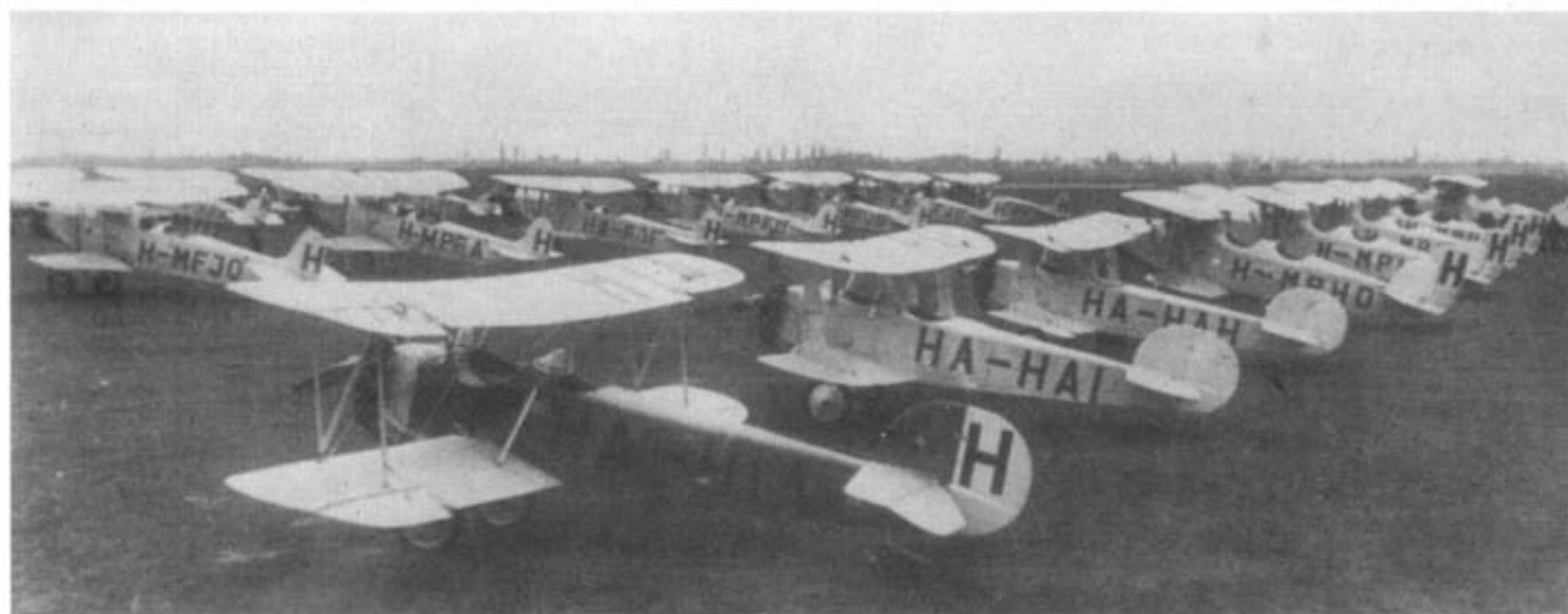
Aircraft of the secret Hungarian air force. Nearest row includes two variants of Hungárias and some Heinkel HD-22s. The second and third rows include Fokker CVs and Heinkel HD-22s. Each unit was given a cover name; for example: "Meteorological Air Agency of the Ministry of Commerce". (Photo: via Ferenc Kovács)
