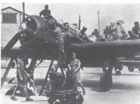
1 The 1,010 h.p. Bristol Pegasus XXII of Wellesley L2637, the first of five converted for the Long Range Development Unit (LRDU) during ground-running tests at Brooklands, February 18, 1938. (All photos: Vickers unless otherwise stated)
