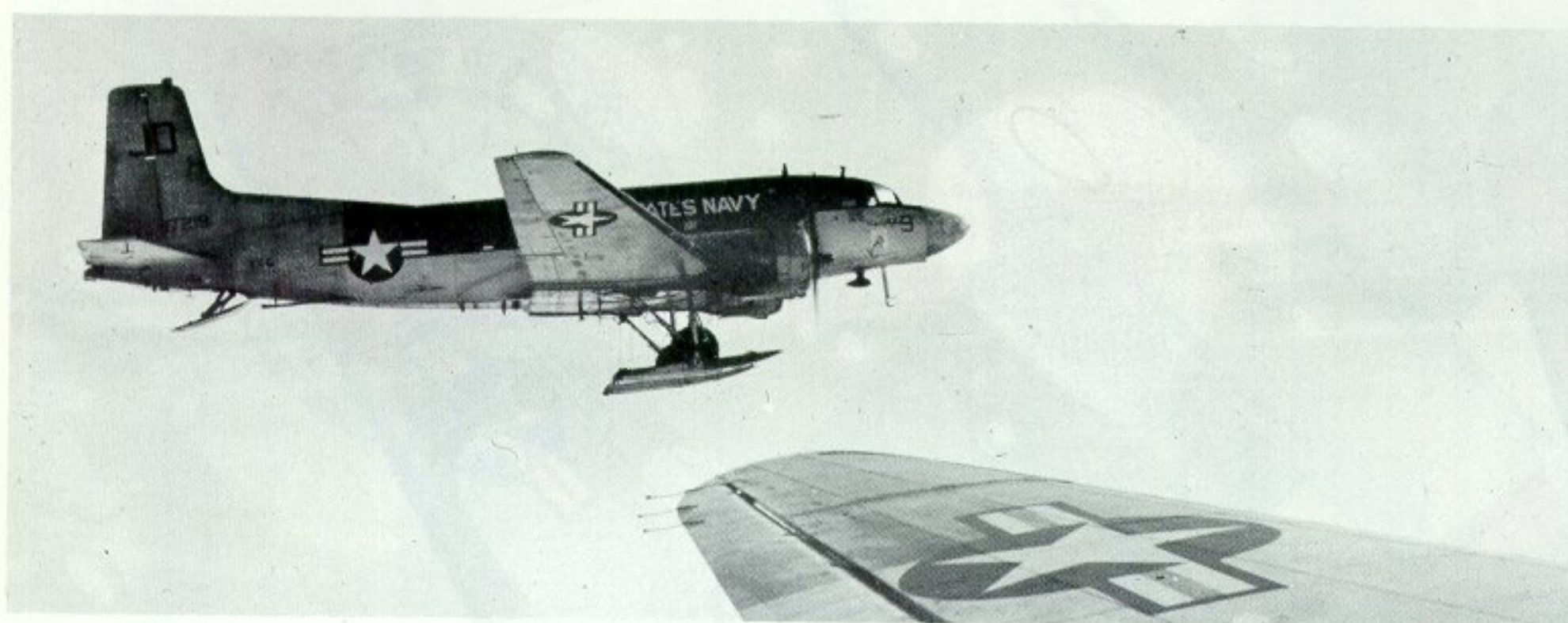
Seen at Detroit, Michigan during April 1956 this R4D-6S (BuNo. 99840) is from VX-1 (Experimental) Squadron. Note the 'thimble' radar nose and tail probe. (Photo: Bill Balogh)
