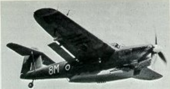
BV727, a Blackburn-built Barracuda II of the Naval Air-Sea Warfare Development Unit, seen during trials with the Airborne Lifeboat adapted for carriage by the Barracuda. The trials were entirely successful and the lifeboat was put into limited production, for carriage by either the Barracuda II or the Barracuda III.
