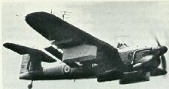
Some mystery surrounds this Barracuda trials installation. Hitherto, it has been described as an "agent" dropper, but as trials did not commence until most of western Europe had been liberated, it is considered more probable that this is the air-portable Naval W/T Station test-flown on a Barracuda II at the beginning of 1945. The aircraft is P9795/G.
