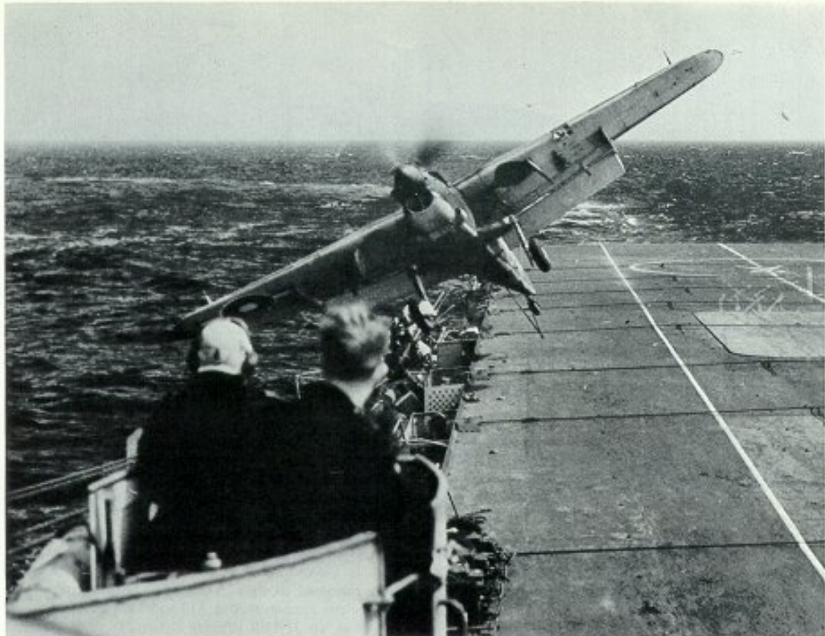
An 814 Squadron Barracuda overshoots to starboard, a hazardous manoeuvre—after the pilot has badly misjudged his circuit, possibly because Venerable steadied on the flying course earlier than he had expected. By the autumn of 1945, the Barracuda squadrons in the Pacific had removed the ASV IIN antennae and most aircraft had only two or four bomb racks. (Photo: Imperial War Museum, ref. A30652)
