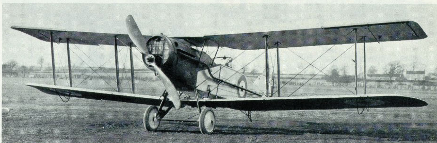
Type 96A, Mk. IIIA (H1417) in March, 1926. This F.2B became the prototype Mk. IV F.2B and had square-cut upper wing tips, due to convenience of affixing wing auto-slots (linked to ailerons). Originally converted to "Mk. II" standard on November 15, 1924; H1417 is seen here with the characteristic Mk. IV larger fin and horn-balanced rudder. (Photo: via C. H. Barnes)
