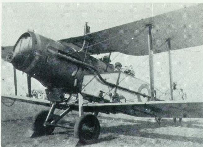
"A" of 28 Squadron preparing for take-off at Secunderabad India, on January 17, 1931. Of particular interest are the "desert" tyres, tropical radiator and upper wing centre-section cooling outlet piping. (Photo: courtesy No. 28 Squadron, RAF)
