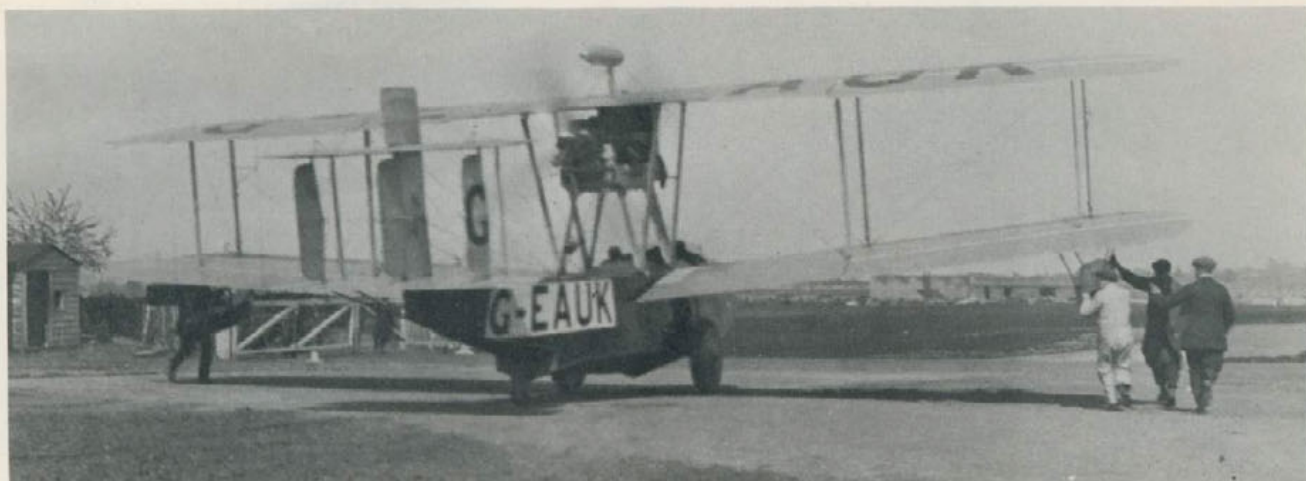
Father: Vickers Type 59 Viking III G-EAUK, seen crossing the railway level crossing at Plough Lane, Croydon, in September 1920 (see page 28). Pilot, Captain S. Cockerell. The slab-sided hard-chine hull contrasts with the more aesthetic roundness of the Seal/Seagull.
