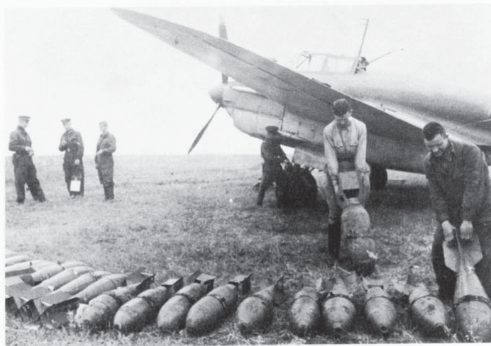
Typical of "in-the-field" operations. In the foreground, an array of 250 kg and the smaller 100 kg bombs. Although an obviously "posed" photograph, the view shows the rear dorsal gun and just reveals the porthole gun position, extreme right.
