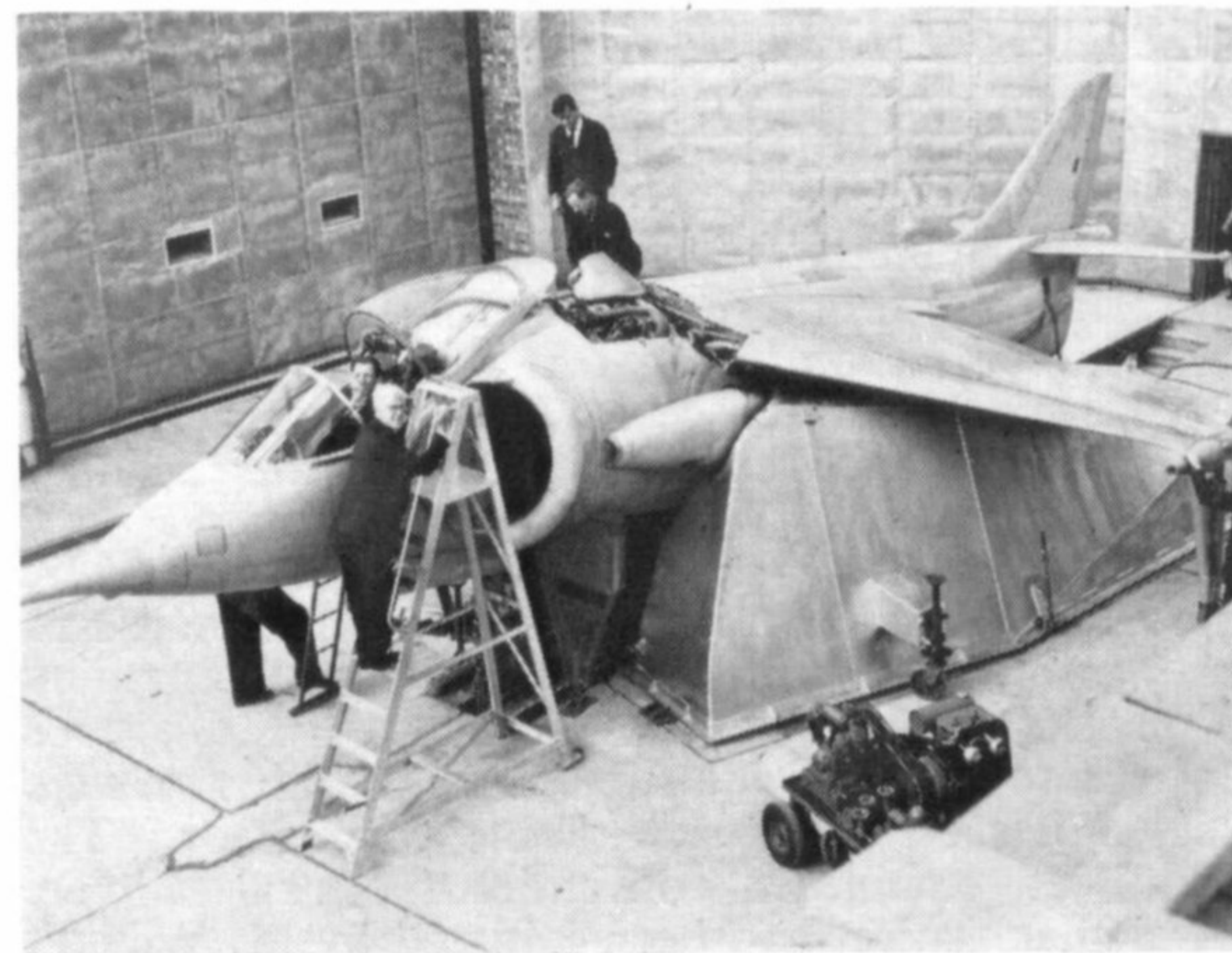
Preparations being made for engine running prior to the first flight. In the cockpit is Bill Bedford, beside him Frank Cross, head of the Experimental Design Office. The large sheet metal shrouds were designed to allow both horizontal and vertical nozzle positions during engine running. (Neg. No. EXP256/60)
