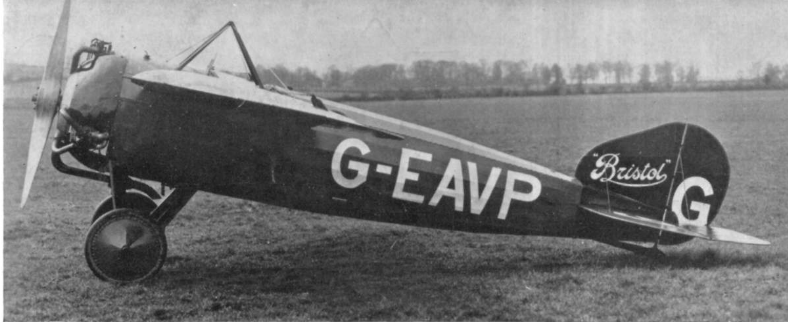
The Bristol M.1D, G-EAVP, a conversion of an M.1B with Bristol Lucifer engine. Comparison of this photograph with that of G-EAVO illustrates the revised shape of the M.1D's fin and rudder.
