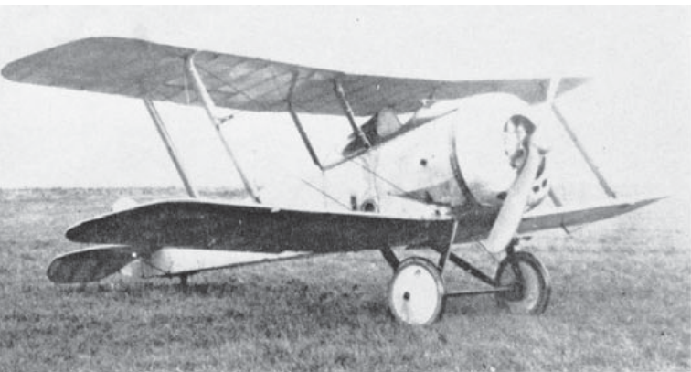
The prototype, still unarmed and with its original fin and rudder, but with a small spinner on the airscrew hub.
