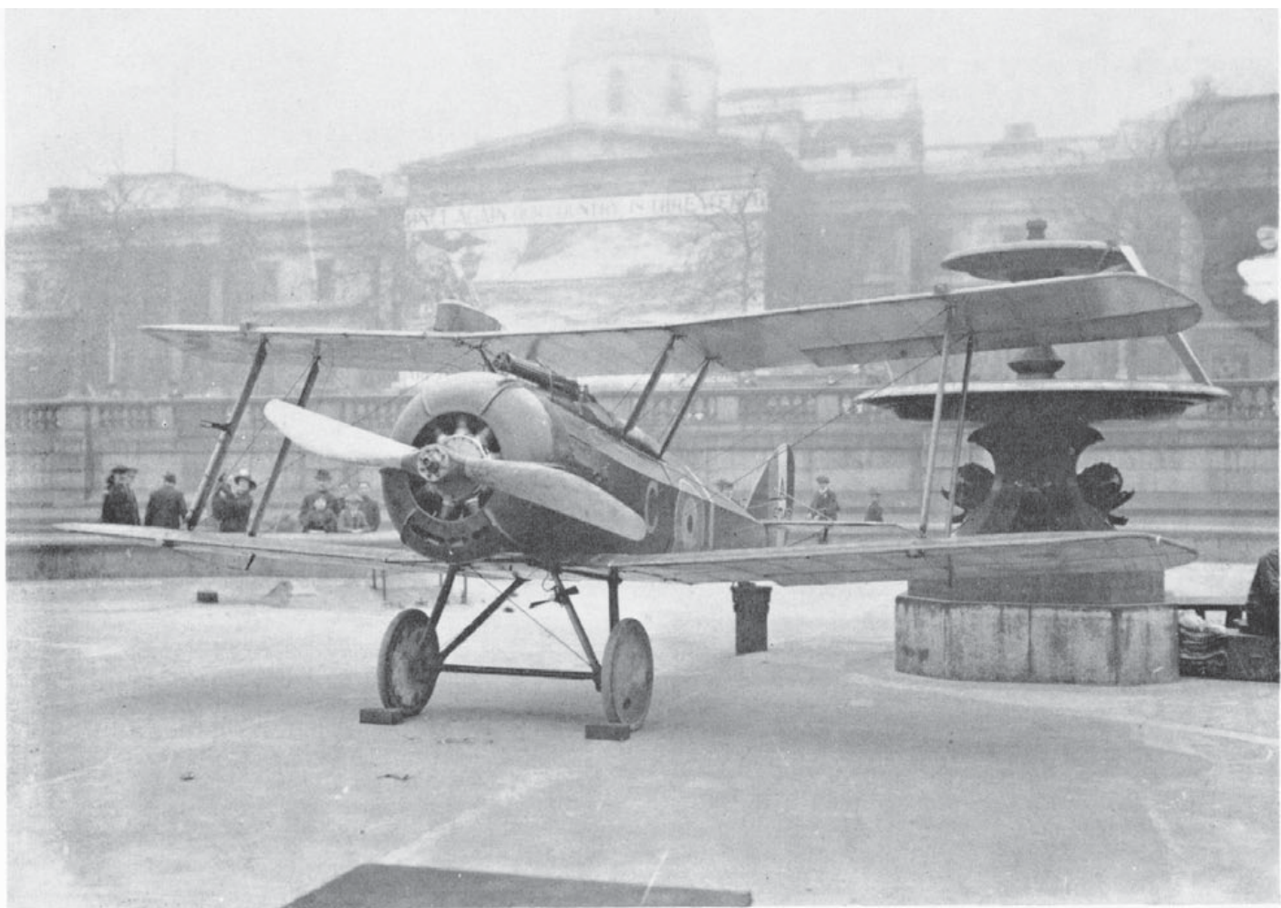
A9340 on display in Trafalgar Square in March 1918 during the Y.M.C.A. Blue Triangle Week. The aircraft seems to have been something of a lash-up for this occasion: the lower starboard wing has a roundel on its upper surface and must originally have been an upper wing on another D.H.5; and the underwing aileron control cables are slack. The markings are those of No. 32 Squadron, R.F.C., but the authenticity of the individual letter C is questionable. (Photos: Flight International 33 and 34)
