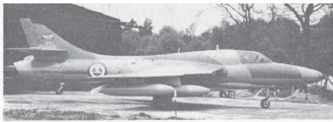
Left: Genuine Hunter T.69 destined for Iraq. (Photo: R. C. B. Ashworth). Right: First Saudi Arabian Hunter T.7 70-616, with four finned 100-gallon drop tanks. (Photo: D. J. Smith, via R. Ward)
