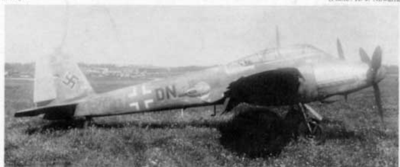
Messerschmitt Me 410A-3, W.Nr.10047, "5T + DN" of an unidentified reconnaissance unit. It will be noticed that the cowling, barbettes, cockpit framing and rudder are still in bare metal finish, possibly indicating replacement parts hastily fitted to a damaged aircraft. (Photo: H. J. Nowarra)
