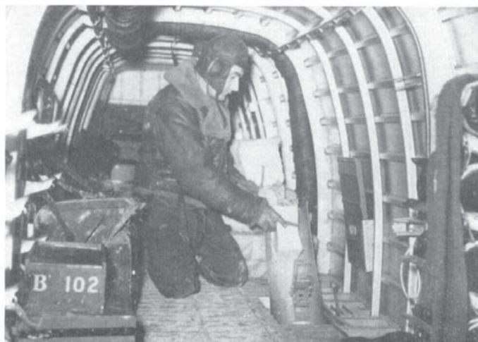
Crew member of No. 102 Squadron's Whitley V "B-Baker" demonstrates how " Nickels " were dropped down flare chute. (Photo: Imperial War Museum)
