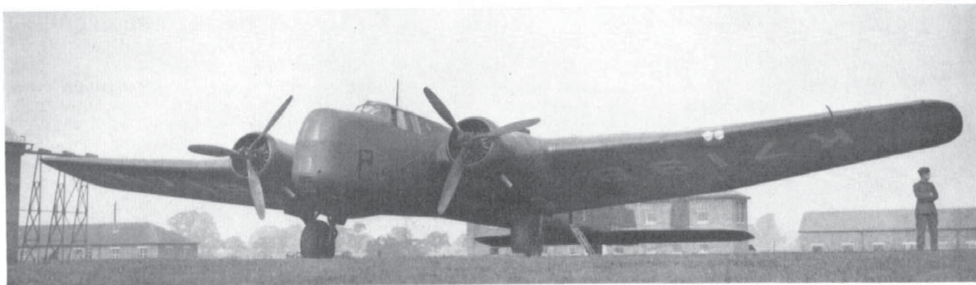
First Whitley Squadron was No. 10, one of whose Mk. I's (K7199 "P-Peter") is shown above. Early Whitleys often lacked nose armament at first, turrets being fitted eventually by Messrs. Airwork at Heston. Below: Mk. IV K9024 sporting No. 10 Squadron's badge on its nose.
