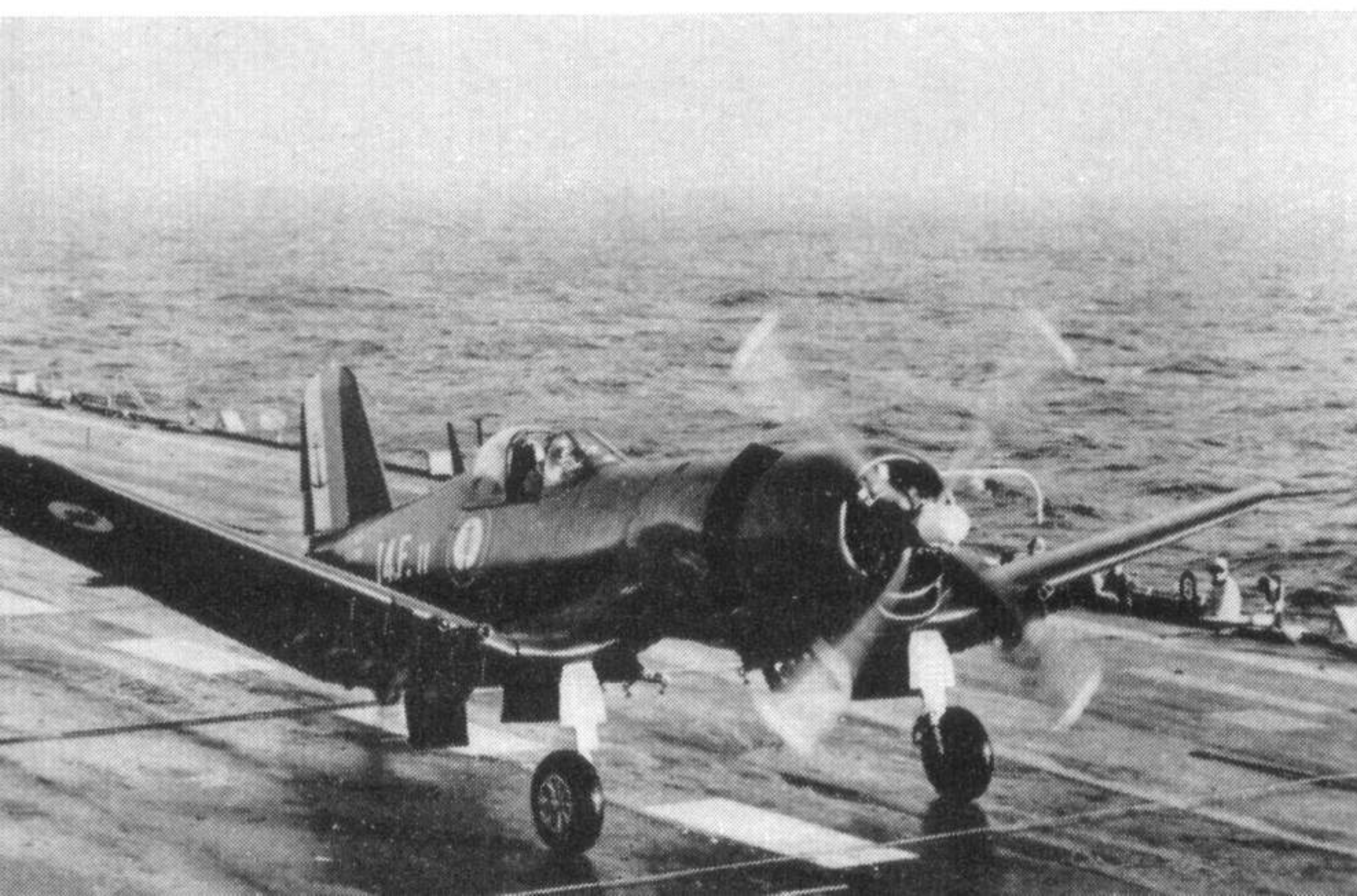
Early rounded windshield on a Korea-based F4U-4.
