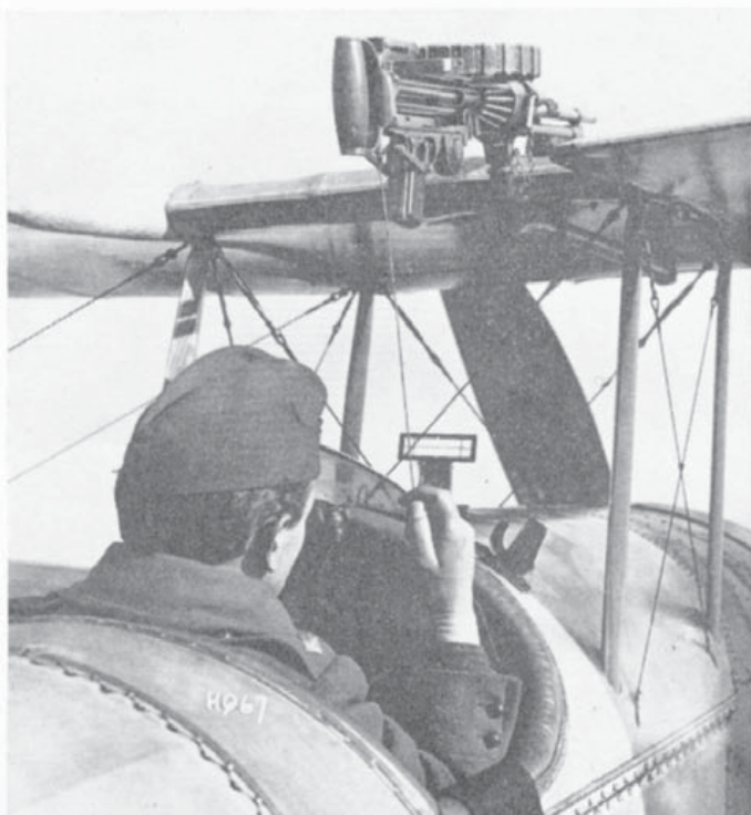
Overwing mounting of Lewis gun on R.F.C. Scout C. The gun was held in the level and vertical positions by spring clips, and the firing control was somewhat primitive. An unusual gun sight is fitted.
