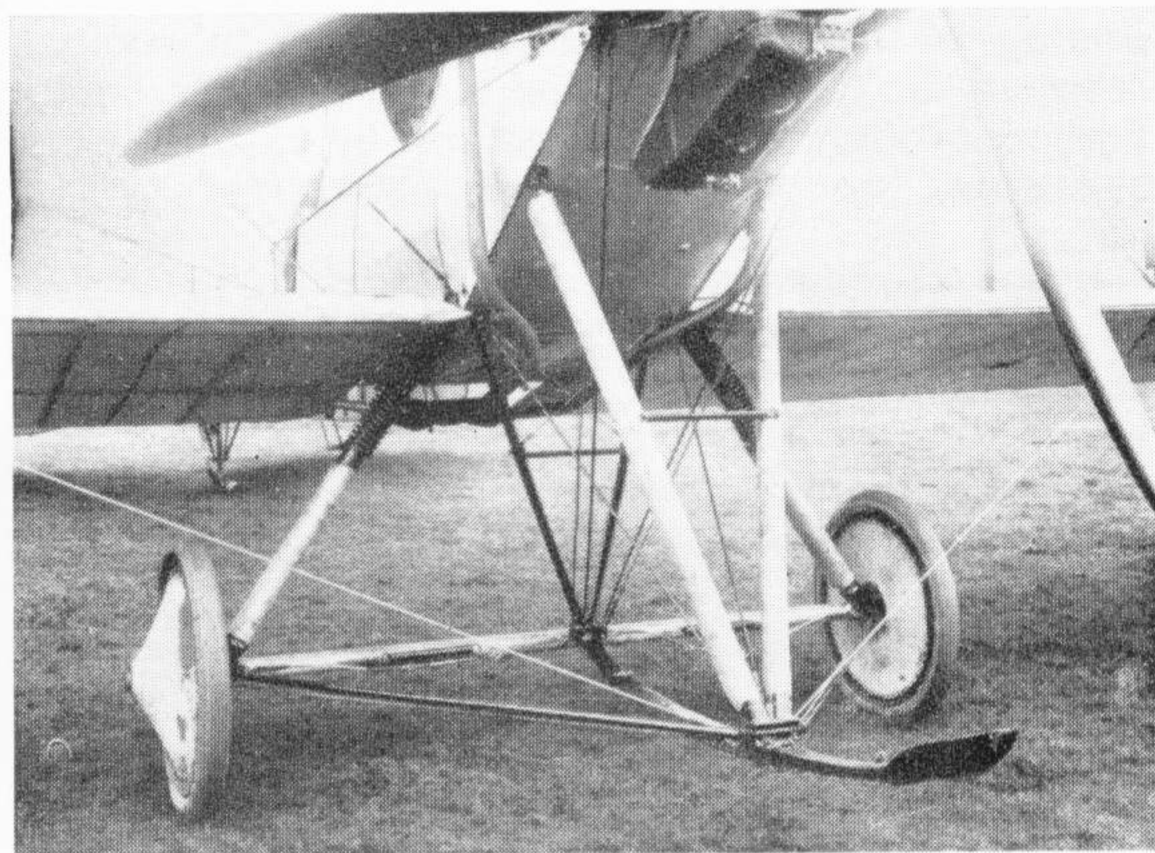
Left: The oleo undercarriage fitted to this B.E.2a was basically that which was later fitted to the F.E.2a, 2b, 2c, 2d, R.E.7 and some B.E.2c's. Photograph dated 11th December 1913. Right: Also dated 11th December 1913, this photograph depicts another form of oleo undercarriage fitted to a B.E.2a. (Photos: Crown copyright)
