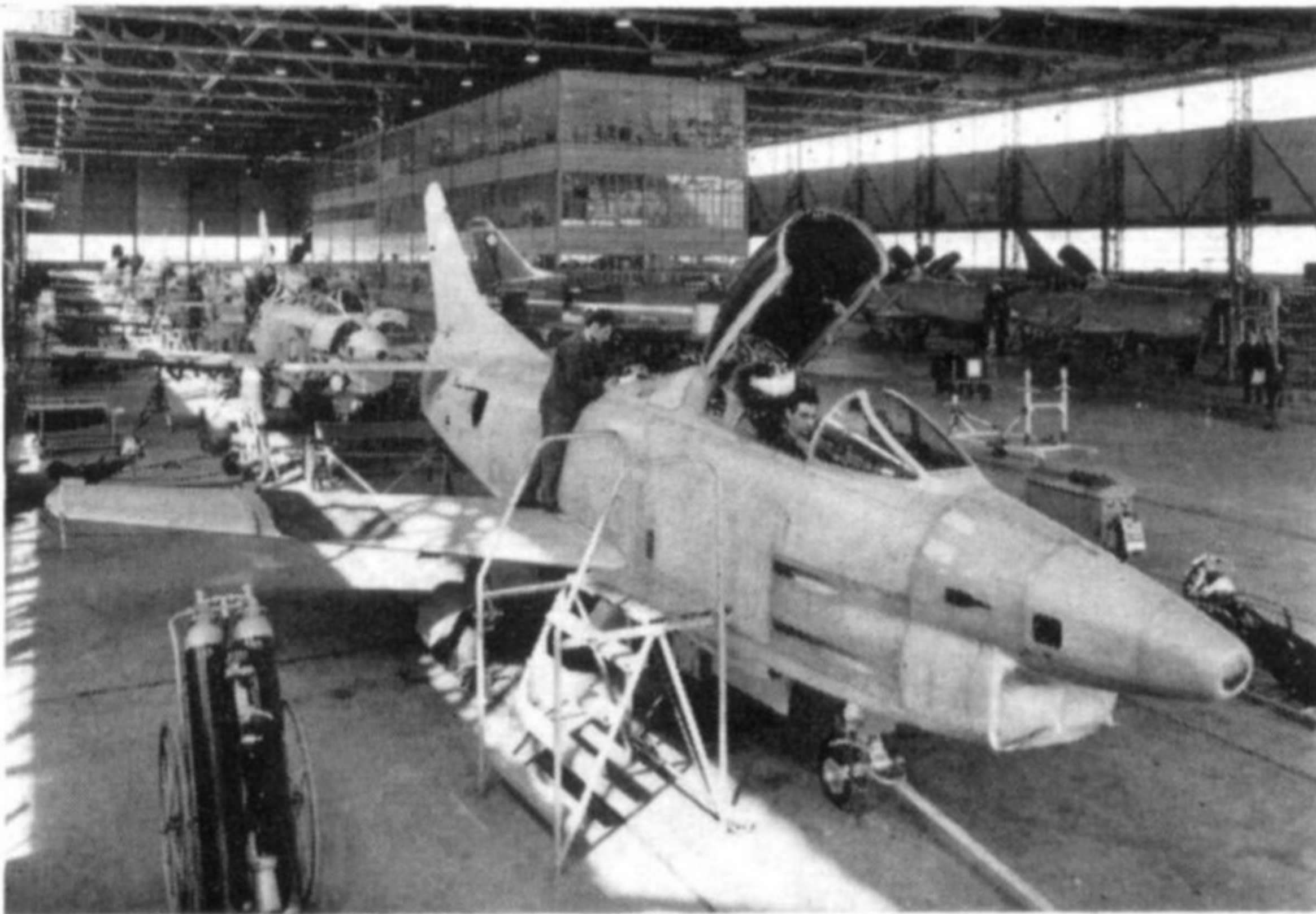
The Fiat plant's G.91 final assembly line. (Photo: Fiat).
