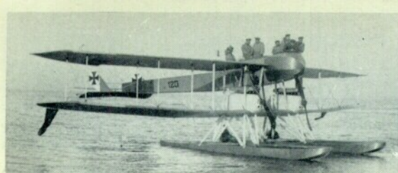
Gotha UWD, the seaplane version of the G.I. Note the black German Navy identification streamers on the wingtips. UWD indicated Ursinus Wasser Doppeldecker, Ursinus Sea Biplane. (Photo: E. Krüger)
