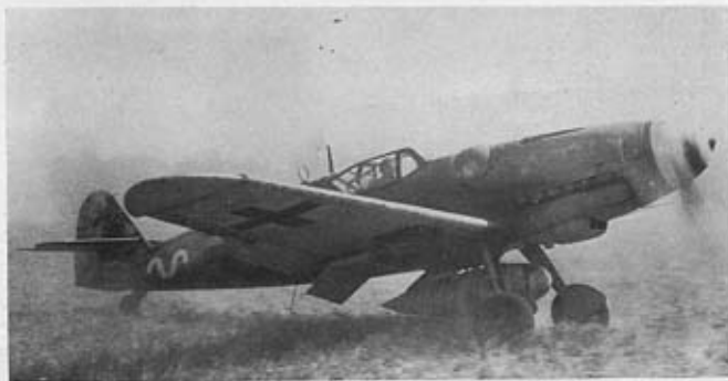
A late-model Bf 109G, probably a G-14, displays the tall tail and the clear-view Gullard hood of the later variants. Cockpit canopy framing was severely reduced, and the armour plate behind the pilot's head replaced by a frame of bullet-proof glass. Note that although this photograph could not have been taken earlier than 1944, the early-style III Gruppe marking is still carried.
