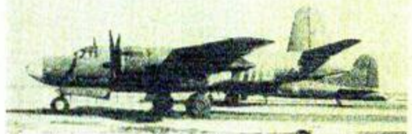
109 machines powered by the R-2800-39 Wasp were delivered as the B-26A-1. (Photo: Peter M. Bowers Collection)
