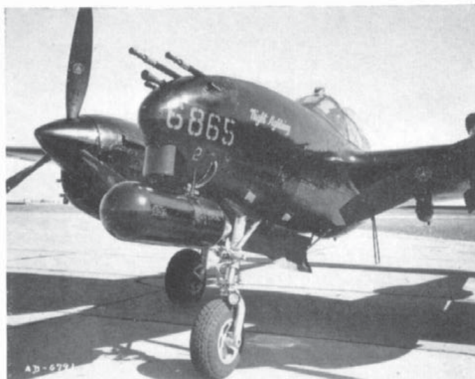
"Night Lightning" (44-26865) the first P-38M night fighter, modified from the P-38L-LO variant. Note A.S.H. radar in "bomb" housing. (Photo: Lockheed)
