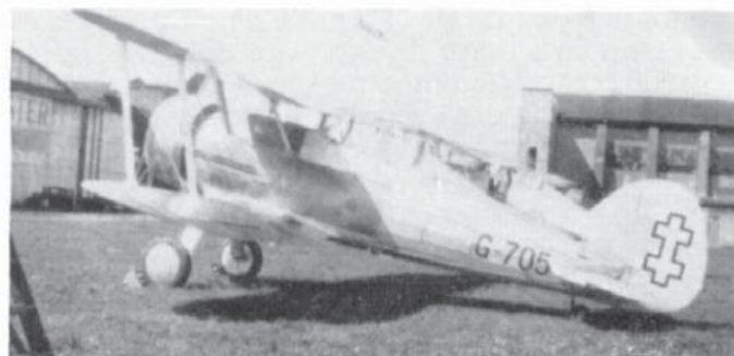
One of 14 Gladiators sold to Lithuania in 1937. Not clearly visible in this view are the upper surfaces which were doped olive drab. (Photo: Bristol Engine Co. Ltd., Neg. No. 18201)
