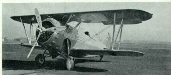
Above: Al Williams' NR1050 Gulfhawk II; highly polished chrome struts combined with brilliant orange finish and blue and white trim to produce an extremely colourful aeroplane. In contrast to other F3F types, the span was 28 ft. 6 in., and the machine had improved spin characteristics. (Photo: Besecker Collection). Below: NC1051 Gulfhawk III is less well known than the single-seater; this G-32 design had split flaps on upper wing. (Photo: Grumman)
