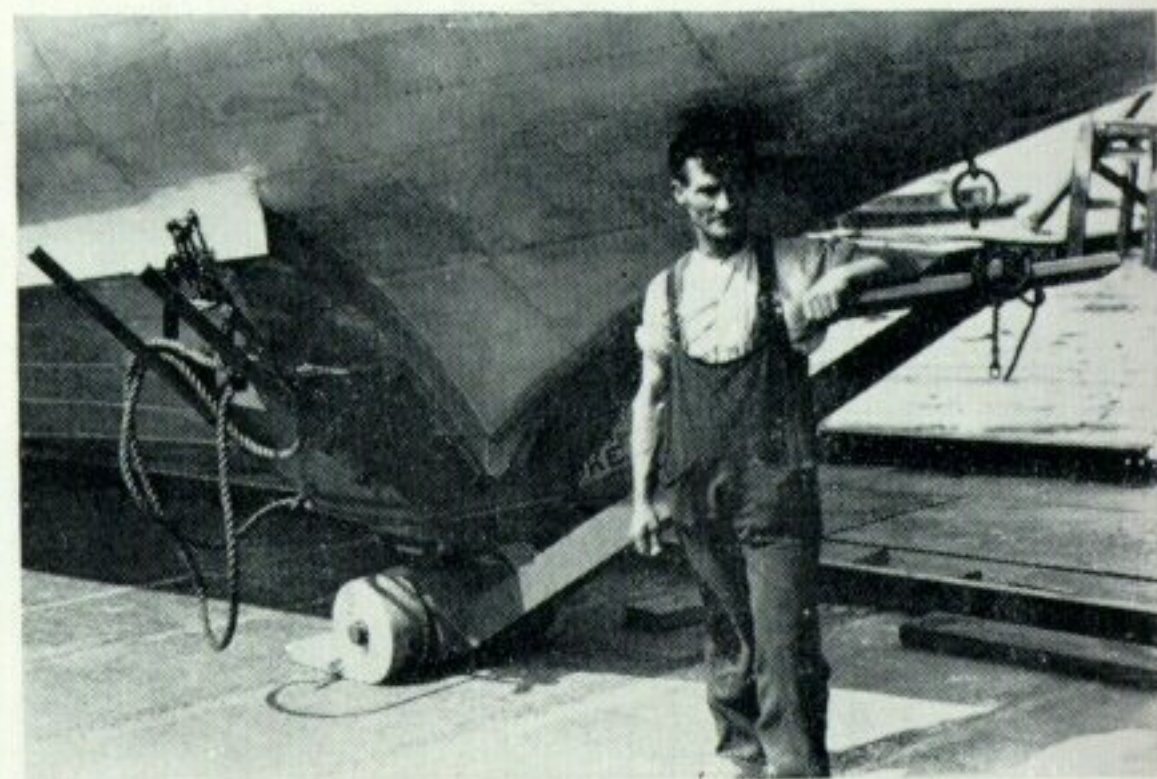
Above and below: Forward and rear beaching gear of Canopus. (Photos: Short Bros. and Harland)
