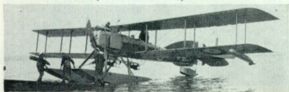
Short Improved 184 N1086 with the original Short-designed Renault installation and lengthened floats, photographed at the Isle of Grain on 1st May 1917.
