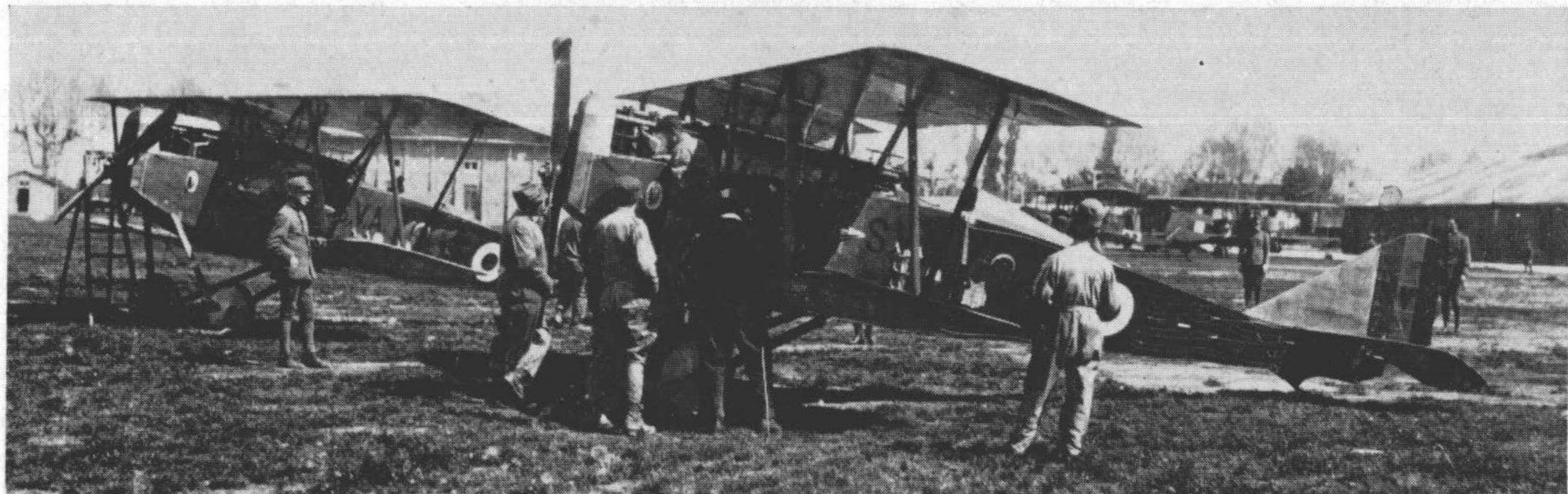
Interesting view of 87° Sq. S.V.A.5s on a forward airfield. The aircraft in the foreground carries three bomb clips on the port side.
