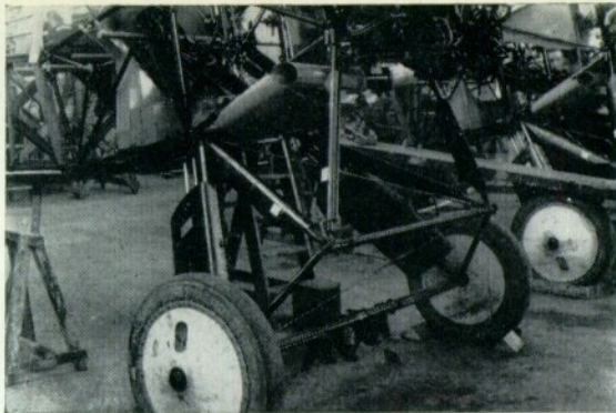
The rugged undercarriage of the Flycatcher: a scene on the production line at Fairey's Hayes factory. (Photo: "Flight")
