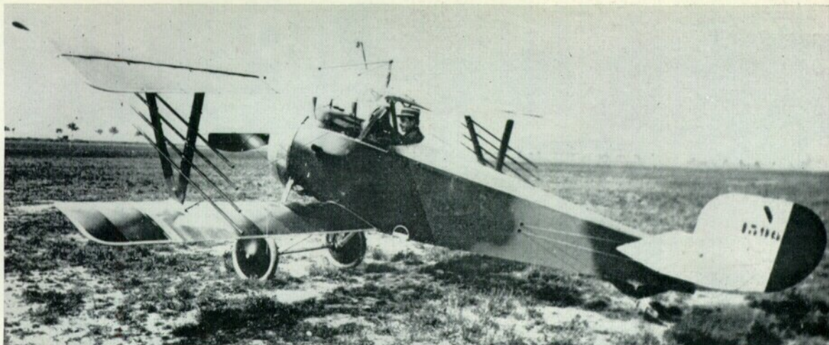
A French Nieuport 17 equipped with Le Prieur incendiary rockets for balloon "bursting".
