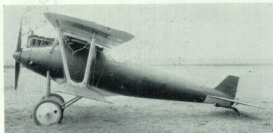
Pfalz D IIIa, 1306/18, landed at Schoondijke, 12th June 1918. In Dutch service until 1920. Note orange disc markings on fuselage and bottom of upper wing. Colour scheme was dark green, with pale blue or silver surfaces. (Photo: G. H. Kamphuis)
