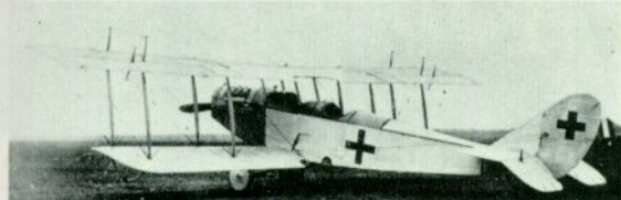
JN-4Ds with special colouring and markings of an Army Ambulance plane. Section behind rear cockpit lifts off to permit insertion of patient on a stretcher.
