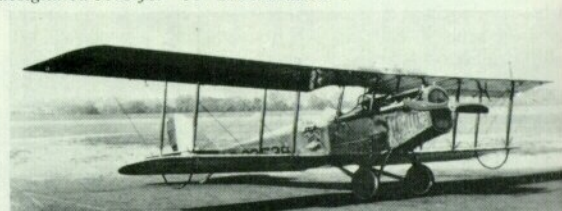
Left: The single JN-5 was a JN-4H modified by the Army to serve as a prototype for the JN-6. Right: JN-4H’s and JN-6H’s rebuilt after W.W.I in U.S. Army depots were redesignated JNS for “JN Standardised”.
