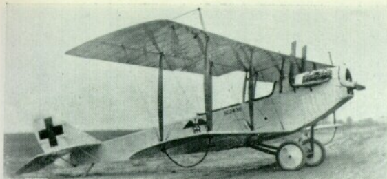
JN-4Ds with special colouring and markings of an Army Ambulance plane. Section behind rear cockpit lifts off to permit insertion of patient on a stretcher.
